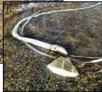
The removal of sediment in a strategically narrowed area deepens and accelerates flows through the cleaned thalweg. Inset: The Sand Wand™ is a manually operated and selectively removes the non-native silts & fine sand material.
