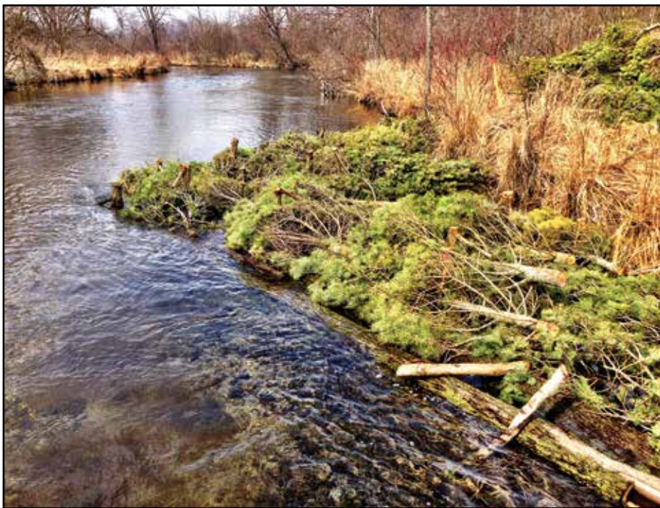
LWD structures are strategically placed in coordination with the sediment deposits left in place to help stabilize depositional areas.
