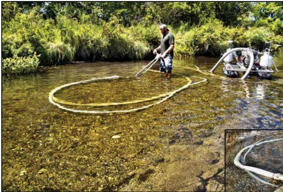
The removal of sediment in a strategically narrowed area deepens and accelerates flows through the cleaned thalweg. Inset: The Sand Wand™ is a manually operated and selectively removes the non-native silts & fine sand material.
