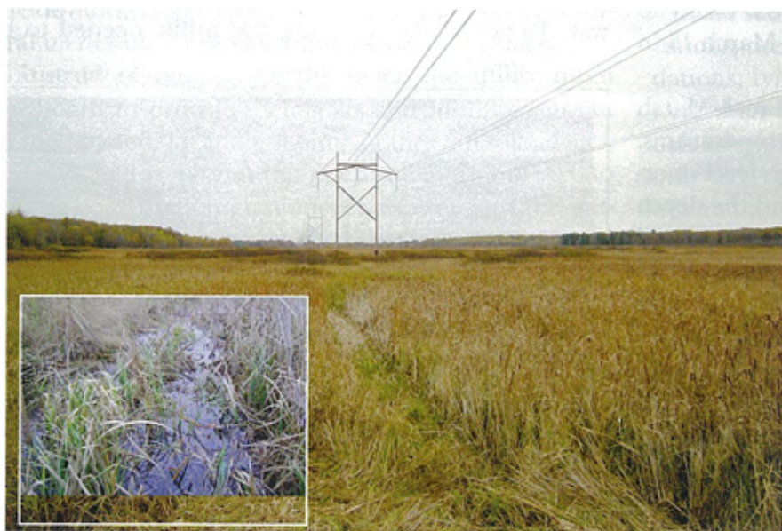
ATC needed access across 5,400 ft of extreme, protected wetlands near Stevens Point, Wisconsin. Traditional wood-mat methods were unable to remedy the problem without adverse environmental impacts and uncontrollable/unpredictable cost. New South's wetlands access experts designed an access road that was built to float on the vegetative layer of the existing marsh. The access road was designed to support 190,000 lbs/36,000-lb axle weight, providing higher weight limits than local paved roads. (Article photos courtesy of New South Equipment Mats.)
